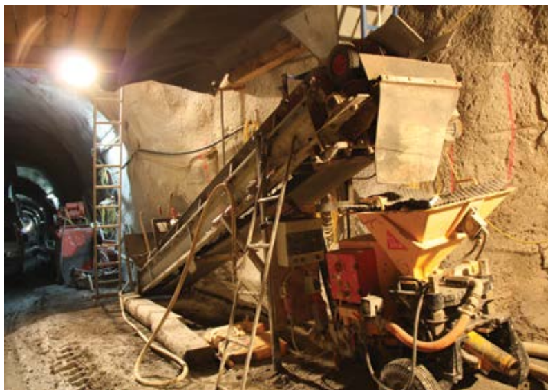
Spraying machine Aliva 257 with on-site conveyer belt
