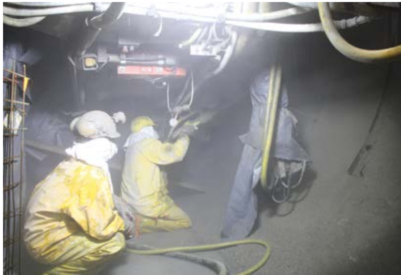
Spraying device for dry-mix shotcrete spraying (behind the drill head)
