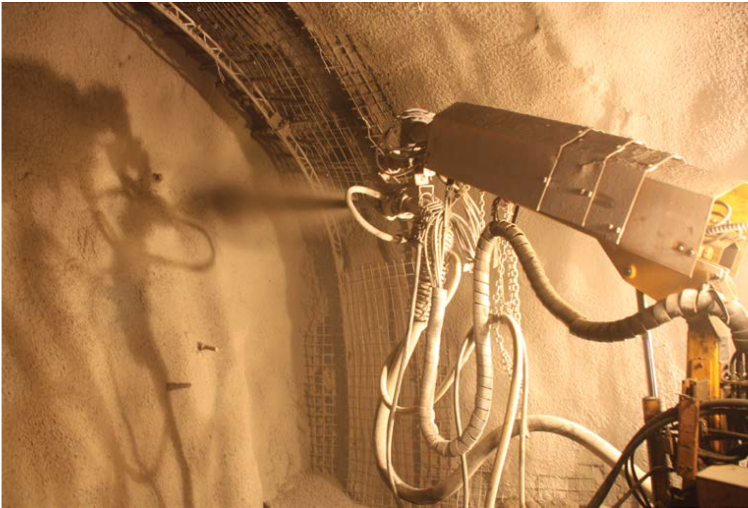
Telescopic spraying arm, Aliva 302. An automatic measurement system was installed into the road tunnel to detect any potential settlements at an early stage
