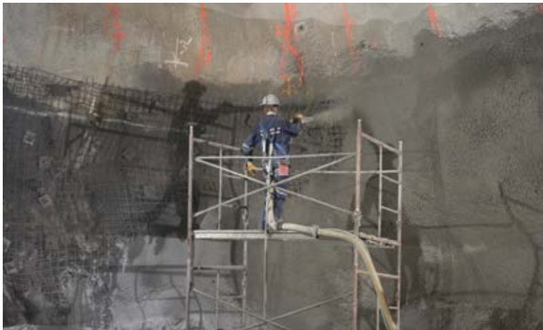
Fig. 1: When placed by an experienced, properly trained crew using well-maintained equipment, dry-mix shotcrete can have minimal effect on the generation of dust
