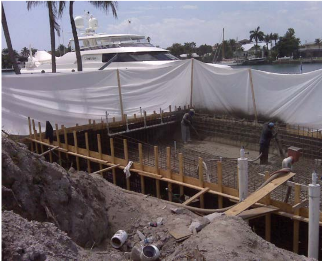
Fig. 1: Typical formwork for pool construction
