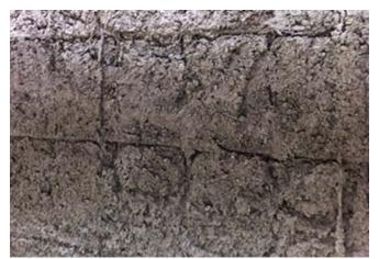
Fig. 2: Uneven flow (slugging) has displaced in-place shotcrete. Note signs of sagging below the wire reinforcement
