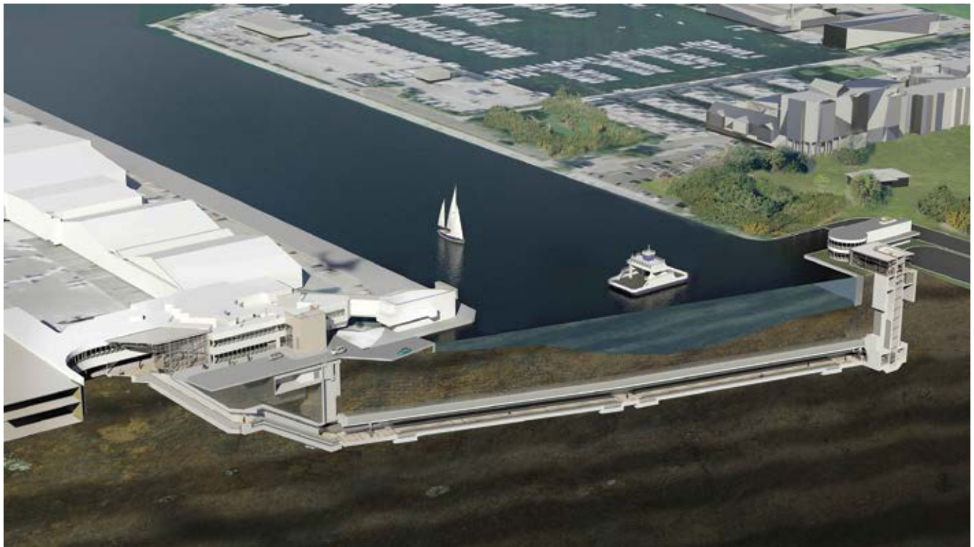
Fig. 4: Three-dimensional cross section of pedestrian walkway. Billy Bishop Toronto City Airport Pedestrian Tunnel Project
