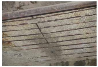
*Fig. 1: Exposed concrete ceiling element has deteriorated beyond its useful service life*
