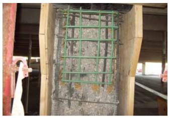
*Fig. 2: The bond characteristic of shotcrete is an important issue for the engineer because it strongly affects repair durability*
