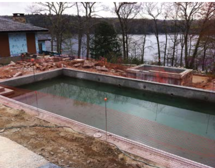
Fig. 2: Pool shell is in place. Ready for the pool deck
