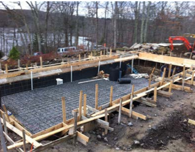
Fig. 1: Lightweight, one-sided form is all that's needed when using shotcrete
