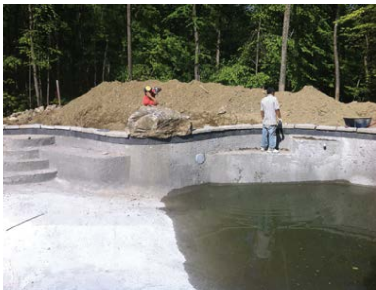
Fig. 4: Using shotcrete makes curved concrete pool surfaces easy
