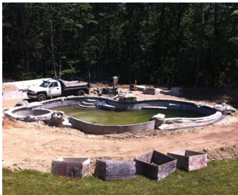
Fig. 3: Overview of a pool with extensive curves typifying shotcrete's flexibility
