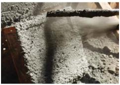
Fig. 3: As the panel fills, the nozzleman adjusts the angle and backs away to avoid displacing in-place material. Note continuous use of a blow pipe
