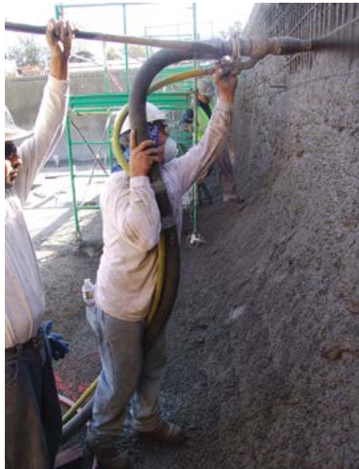
Fig. 2: Nozzleman, air lance man, and finisher in the background
