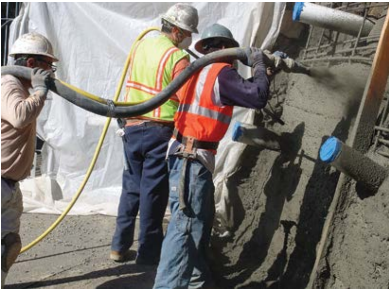
Fig. 1: Nozzleman with his air lance man and hose tender
