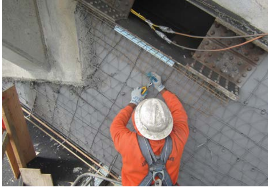
Fig. 4: Repairing mesh prior to shoot
