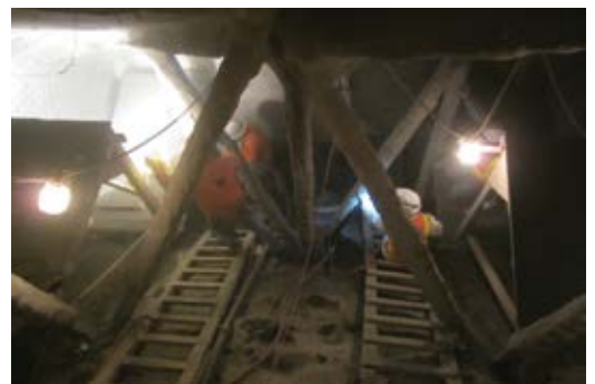
Fig. 2 and 3: Shotcrete placement inside the arches
