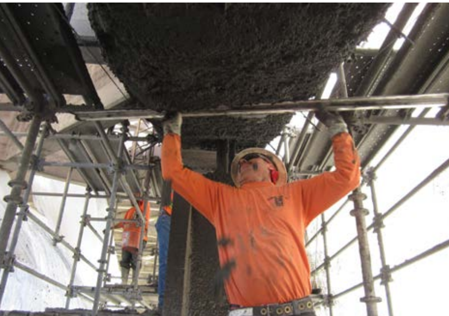
Fig. 8: Overhead finishing
