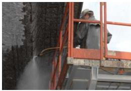
*Fig. 2: High-pressure water blasting the concrete substrate after concrete removal with a jackhammer*
