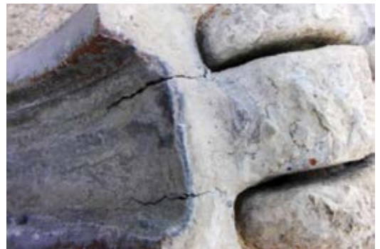
Fig. 2: Daily checklists are a must in preventing injuries. Heavy-duty clamp cracked at the hinge joint
