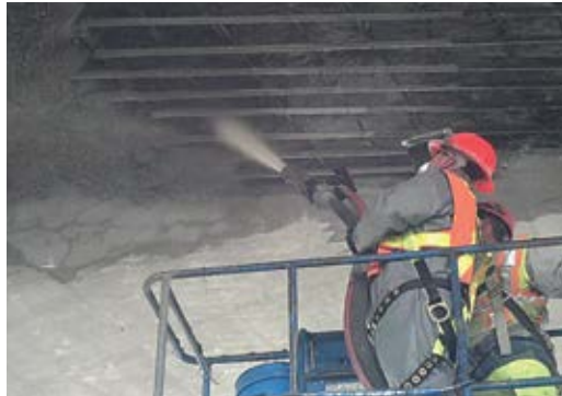
Fig. 9: Nozzleman using anti-static dry-mix hose
