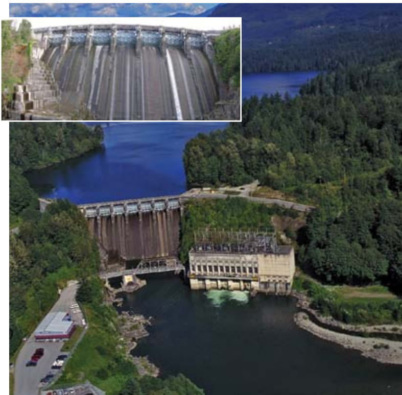
Fig. 1: Ruskin Dam and 105 MW generating station. The spillway (inset) has undergone two renovations in its 80-year life
