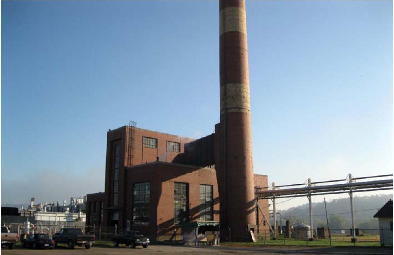
In boilers and other industrial structures, the only access is often through man-doors and up into the boiler or vessel. Shotcrete provides an efficient method of transporting and placing material
