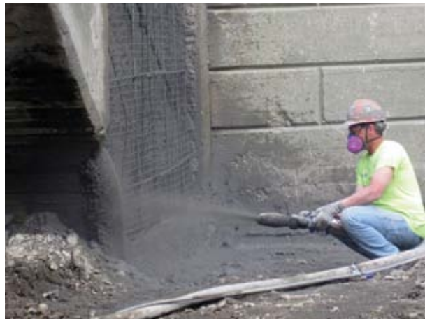
RAM used ACI-certified nozzlemen for all shotcrete placement
