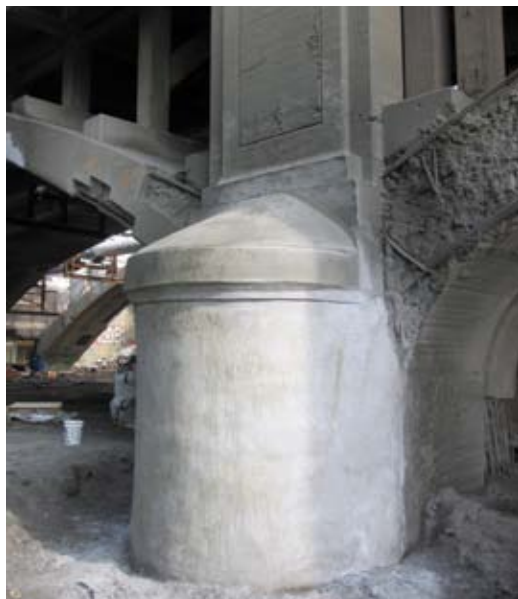
Areas repaired using the dry-mix shotcrete process included bridge piers
