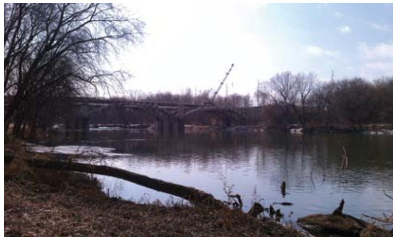
Overview of the Morris Street Bridge project
