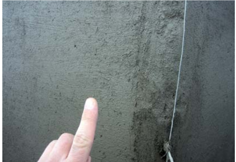
Shotcrete was trowel-finished for aesthetics and also to increase durability
