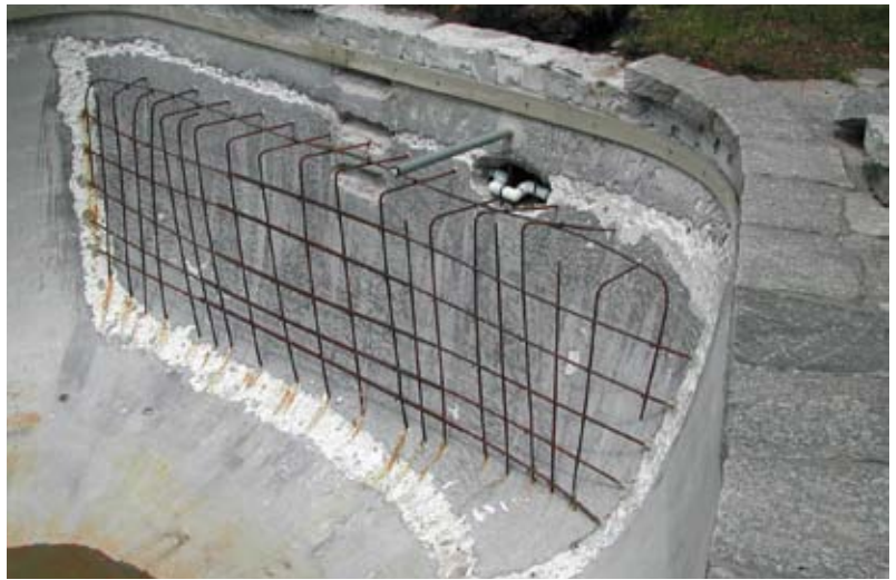
Pool shell ready for shotcrete
