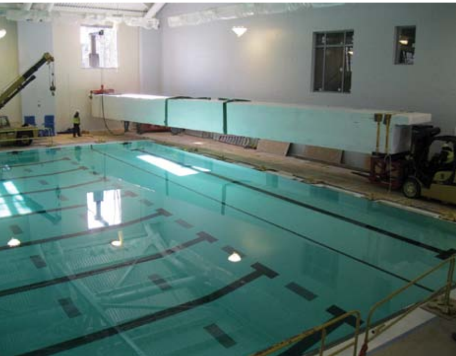
Fig. 1: Installed one of the two bulkheads that go in the pool
