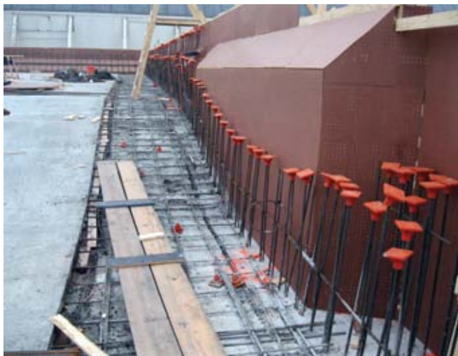
Fig. 2: Pool floor after the floor was cast but before shotcrete placement
