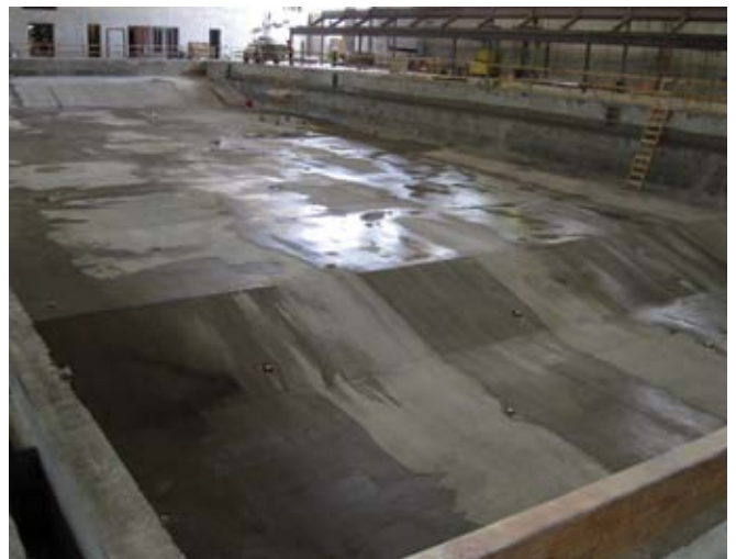
Fig. 3: Completed cast floor and shotcrete walls
