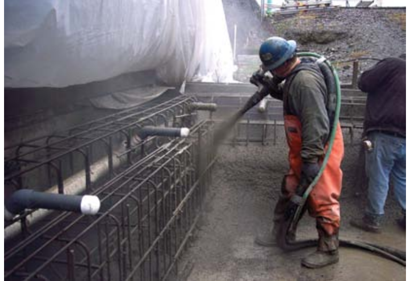
Fig. 6: Wet-mix shotcrete process, ACI Nozzleman shooting base of walls
