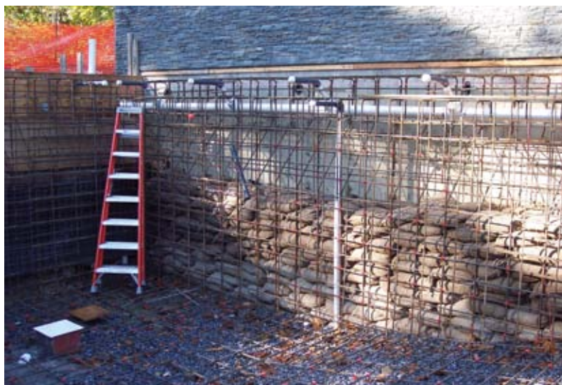
Fig. 4: Reinforcing bar installation, retaining stone bags, and piping
