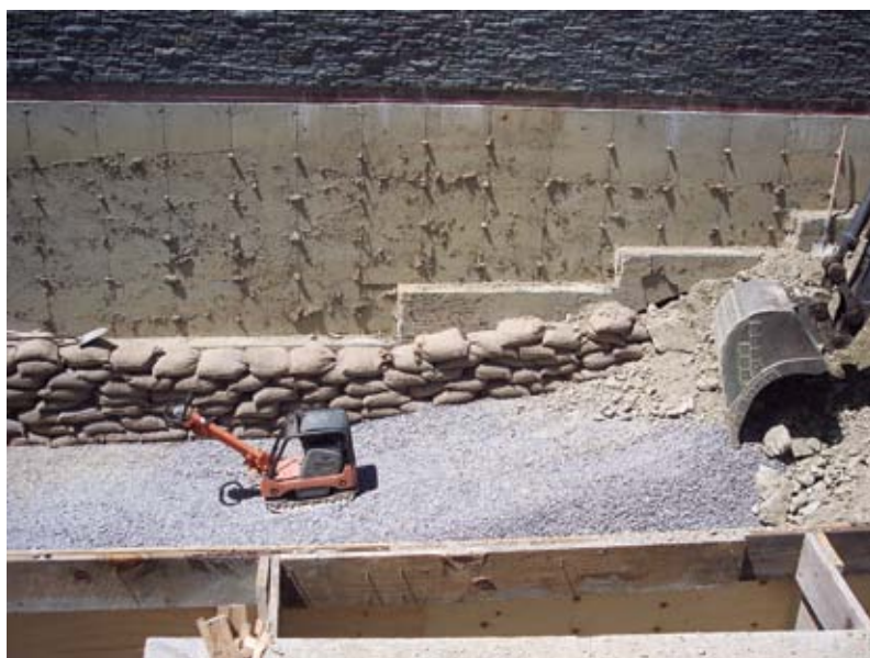
Fig. 3: Drainage stone layer, retaining stone bags, and compaction
