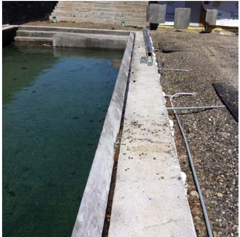
Fig. 7: Lautner edge in place, tank testing for water tightness
