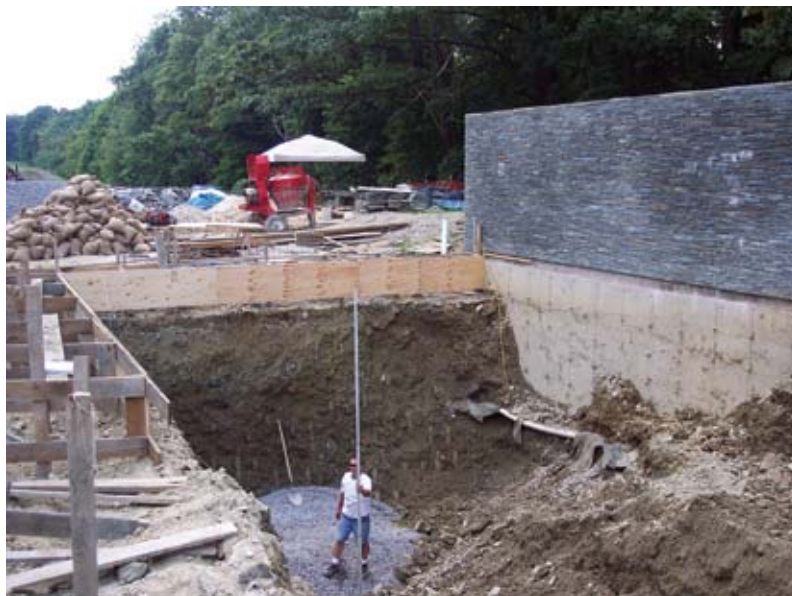
Fig. 2: Bottom of excavation to solid, undisturbed soils/rock
