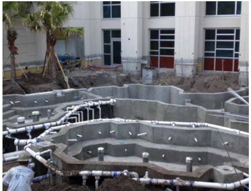
Fig. 6: Spa construction, Peabody Hotel, Orlando, FL
