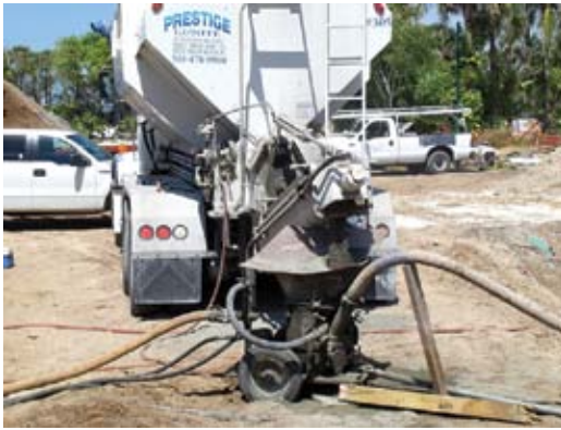
Fig. 4: Batching truck with rotary gun for dry-mix application
