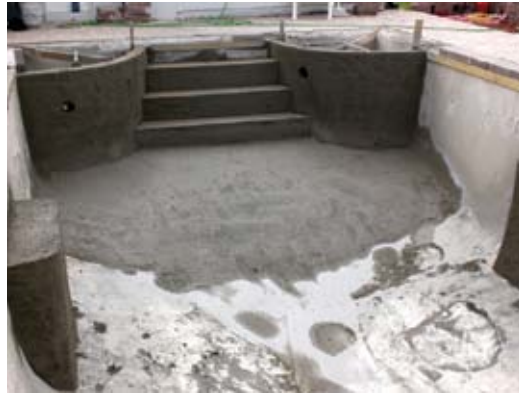
Fig. 8: Dry-mix process used for renovation, adding step and planters
