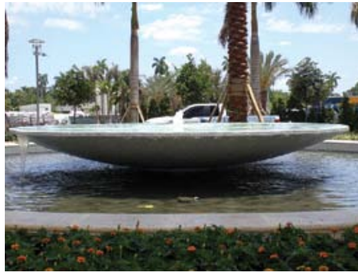
Fig. 9: Dry-mix process used for fountain at a condominium, Ft. Myers, FL
