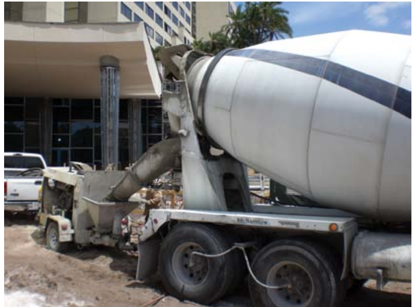
Fig. 5: Wet-mix concrete delivery truck and pump, Peabody Hotel, Orlando, FL
