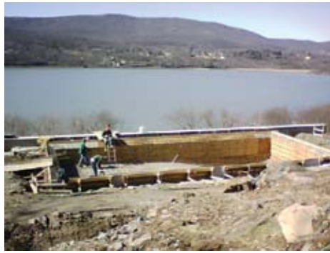
Pool being formed and steeled with one wall as a backdrop
