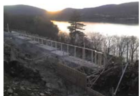
Wall footings with wall forms beginning to be installed
