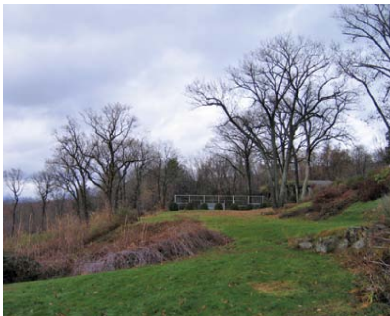
Property before pool and wall construction began
