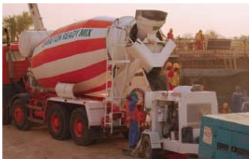
Fig. 1: Concrete supply by UNIBETON Ready Mix
