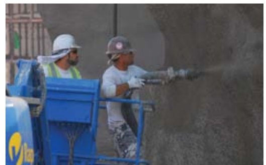
Fig. 2: Shotcreting by Imagineering
