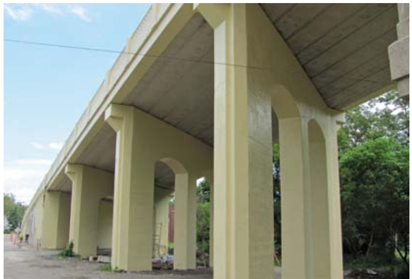
Fig. 3: Rehabilitated columns with tintable epoxy urethane sealer
