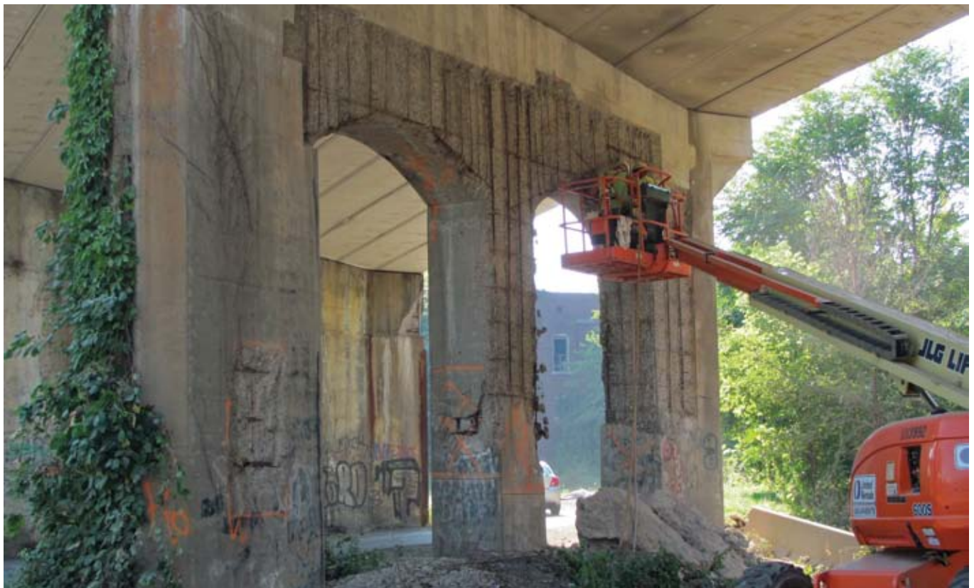
Fig. 1: Deteriorated concrete being removed during demolition
