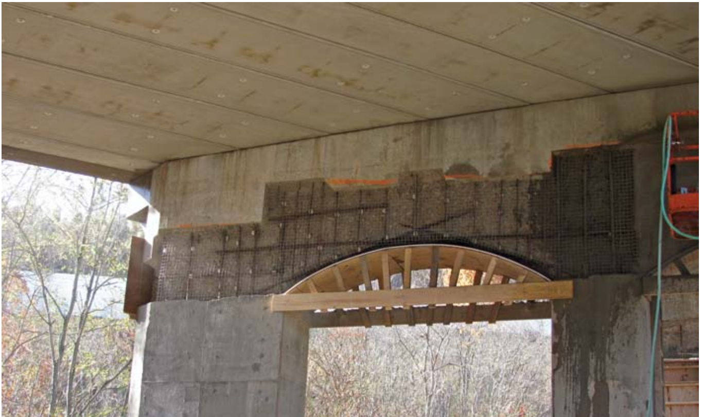
Fig. 2: Wire mesh and anodes installed prior to material installation
