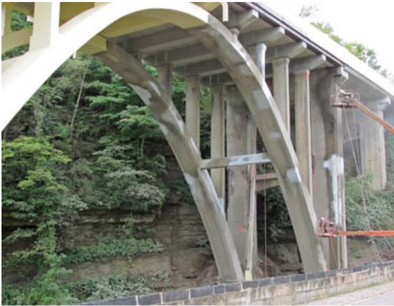
Fig. 4: Open spandrel arch and spandrel column rehabilitation
