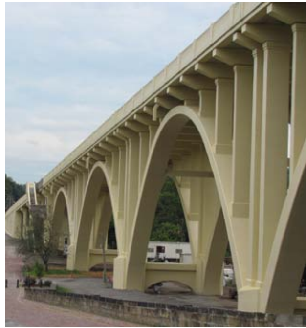
Fig. 5: Rehabilitation of Blaine Hill Viaduct Bridge near completion
