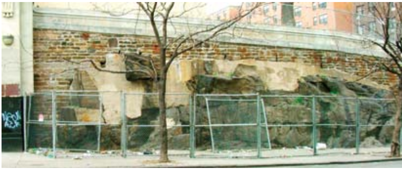
Fig. 3: Drilling rock anchor borehole
