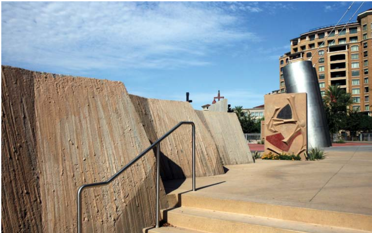
Drip method and earth-cast wall
