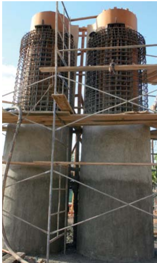
Anchor pylons shot using a template
