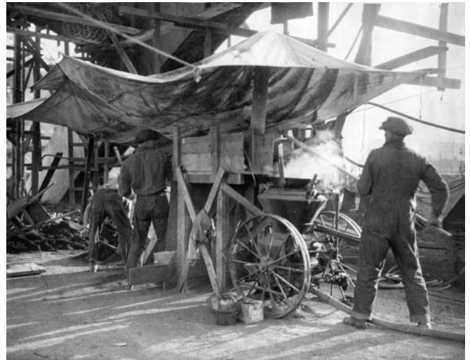
Oregon City Bridge during construction Photo courtesy of the Oregon Department of Transportation
