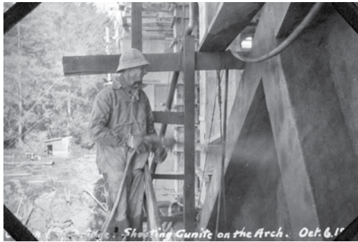
Oregon City Bridge during construction
