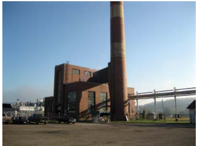
Fig. 3: Shotcrete provides a fast, efficient method of installing refractory in power plants and other industrial applications under difficult time constraints
