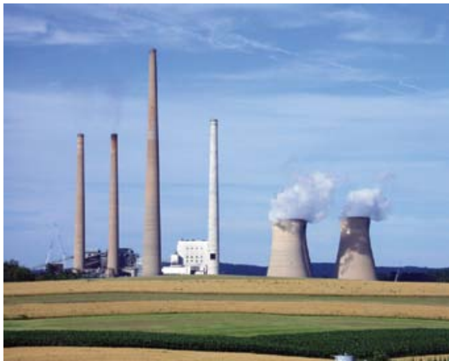
Fig. 1: In plant outage work, at facilities such as the Homer City Generating Station pictured here, shotcrete can provide an efficient method of installing refractory
