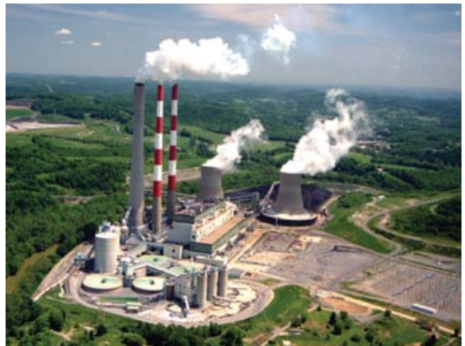
Fig. 2: Lost production time at large power plants, such as the Harrison Power Station pictured here, can be extremely expensive and repair work must be compressed into the time allotted in the scheduled outage
