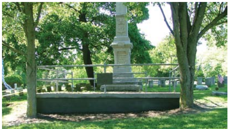
Fig. 5: Completed shotcrete placement on the monument review stand
