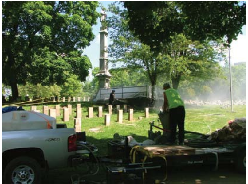
Fig. 3: Overview of the site with the dry-mix rig in the foreground
