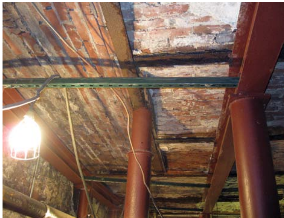
Fig. 4: The general condition and configuration of the brick arches. There were also places with holes or missing bricks
