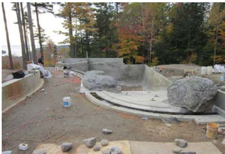
Fig. 4: Completed shotcrete with large rocks placed
