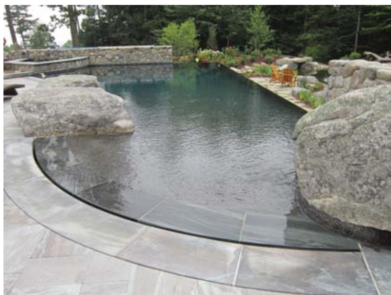
Fig. 5: Completed pool from the beach-entry end
