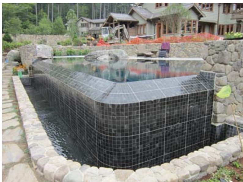
Fig. 6: Completed pool from the negative-edge side
