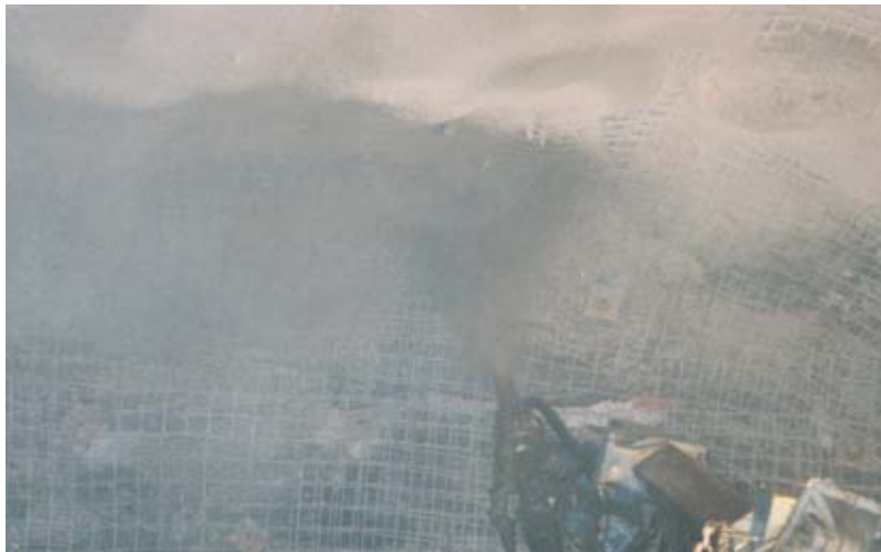
Fig. 1: Sprayer operator spraying the roof before the walls
