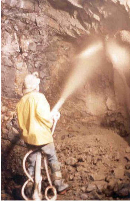
Fig. 3: Even some hand nozzling is improperly sequenced
