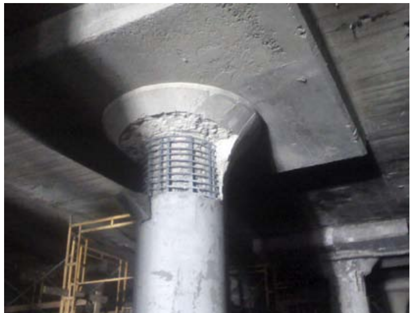
Fig. 5: Column prepared for shotcrete application
