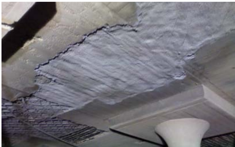
Fig. 6: Multiple layers of shotcrete prior to finish coat
