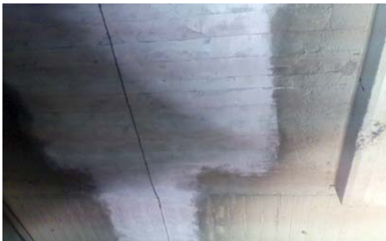
Fig. 7: New shotcrete surface to resemble 1932-formed rough-cut plank finish
