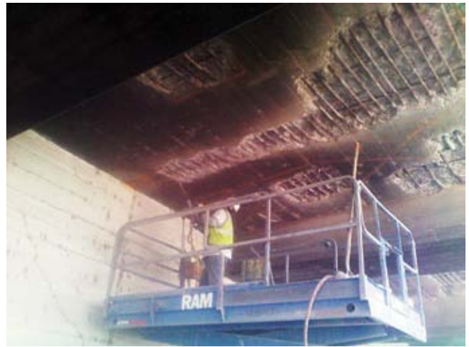
Fig. 3: Smaller, isolated concrete repairs manually removed by a pneumatic jackhammer
