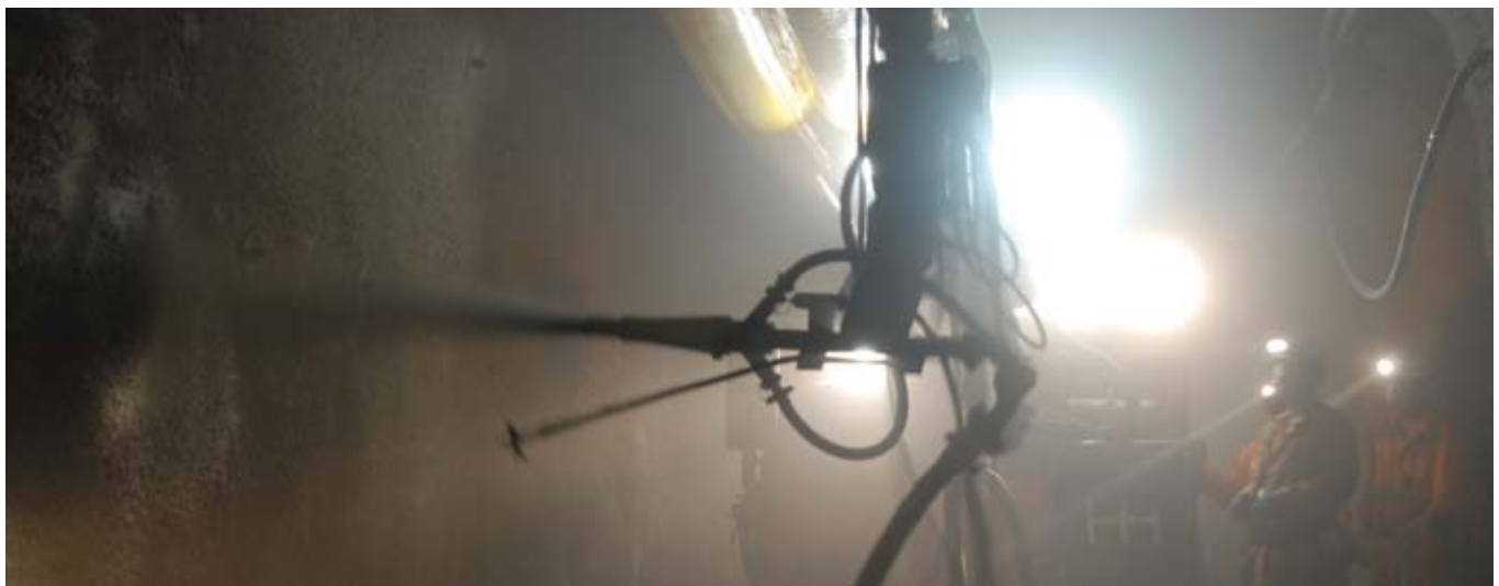
Fig. 1: Once the shotcrete has hardened, will its creep characteristics suit the degree of ground movement expected?
