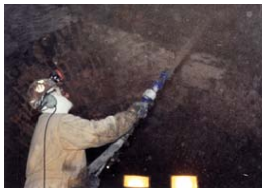
Fig. 5: Shotcrete being placed
