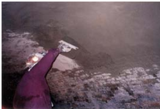
Fig. 6: Shotcrete being cut back to finish grade
