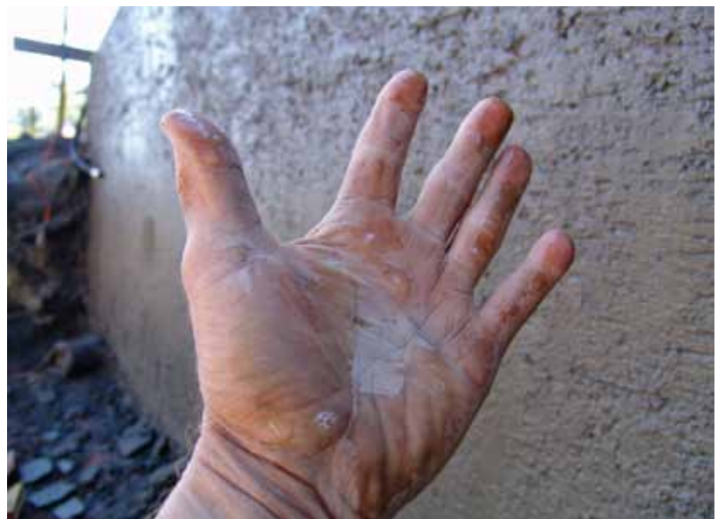
Fig. 3(a): Wall section shortly after saturation. Note its shiny surface; when touched, water is easily transferred to your hand
