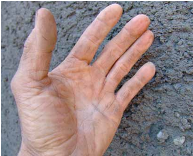
Fig. 3(b): Wall section in surface-dry condition. When touched, water is not transferred to your hand
