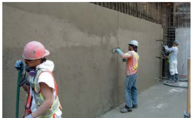
Finishing touches are made to a freshly placed shotcrete wall
