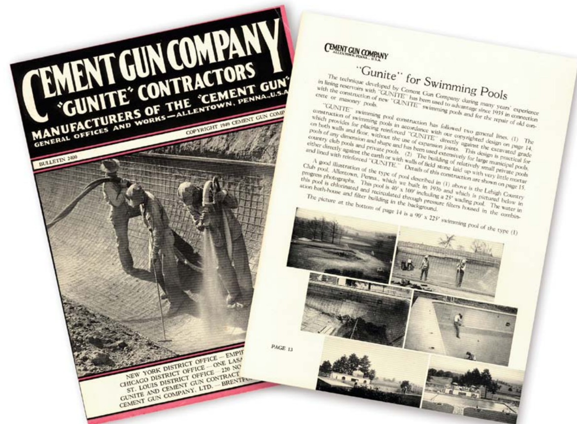
This 1949 publication from the Cement Gun Co. recalls the earliest known use of gunite in the construction of a swimming pool as far back as 1936 in Allentown, PA
