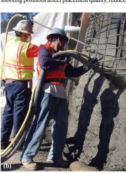
Fig. 3: Examples of awkward nozzle positions. Nozzles held (a) over the shoulder or (b) from the side reduce mobility, range of motion, and overall placement precision
