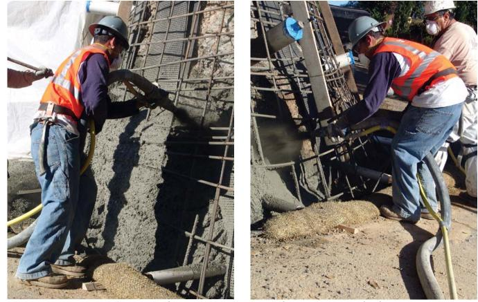
Fig. 6: Expert nozzleman maintains optimum nozzle position at various heights
