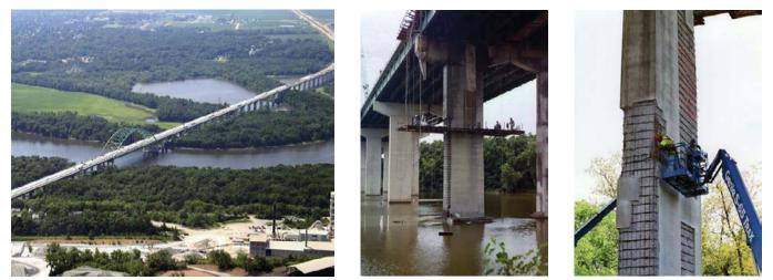
Use of the shotcrete process on the Abraham Memorial Bridge in LaSalle, IL. The contractors chose the shotcrete process following the IDOT "Structural Repair of Concrete" specification
