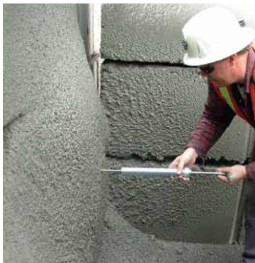
Fig. 4: Using a Proctor penetrometer to gauge initial set
