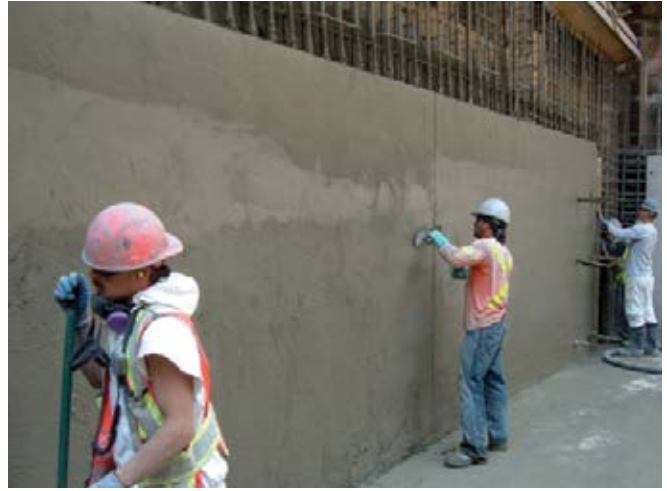
Finishing touches are made to a freshly placed shotcrete wall
