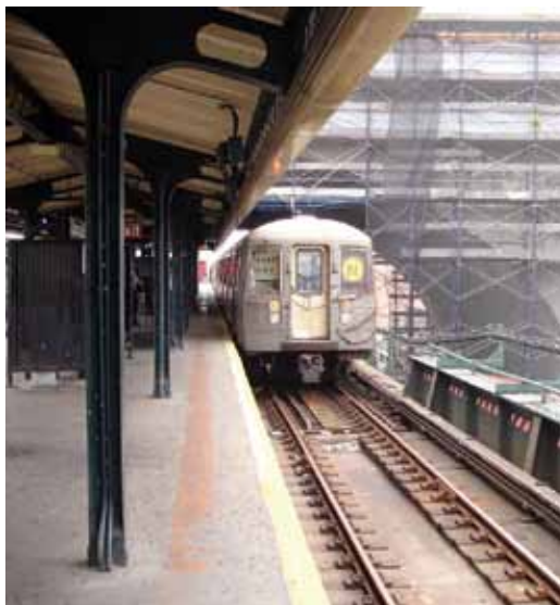
The Ditmars Boulevard Subway Station is partially inside the arched bridge
