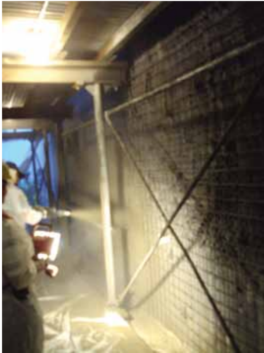
Prepackaged fiber-reinforced wet-mix shotcrete was applied
