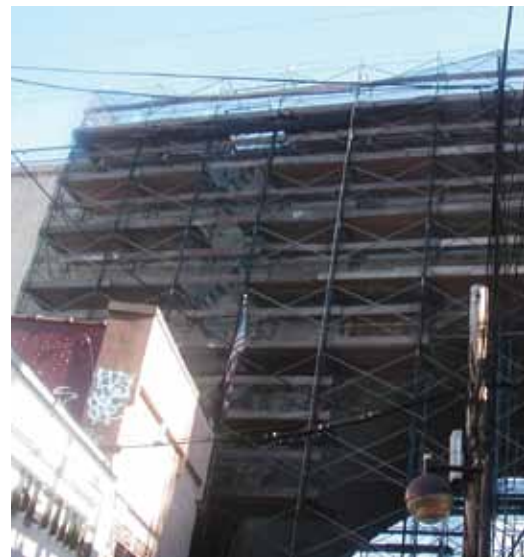
Scaffolds were erected over the elevated subway tracks and 31st Street
