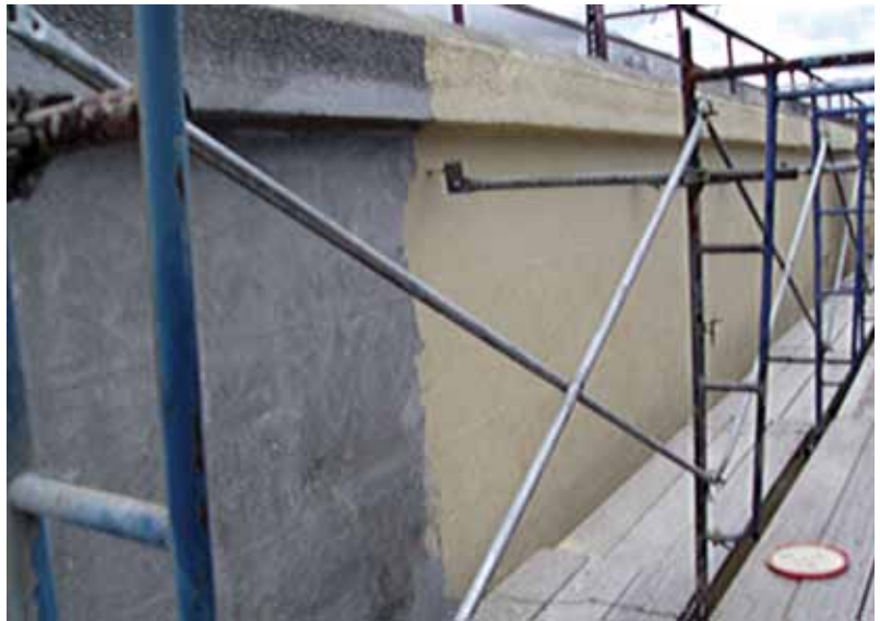
Two coats of a water-dispersed, acrylic, anti-carbonation coating were applied
