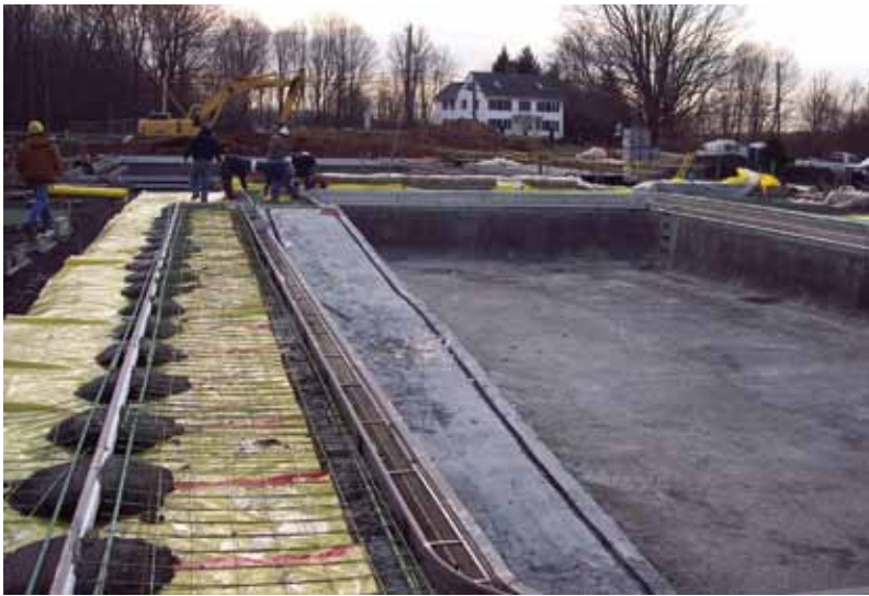
Stainless steel gutter installation
