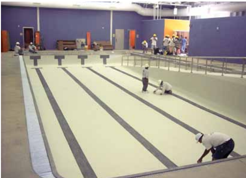
Tested plaster installation over watertight concrete
