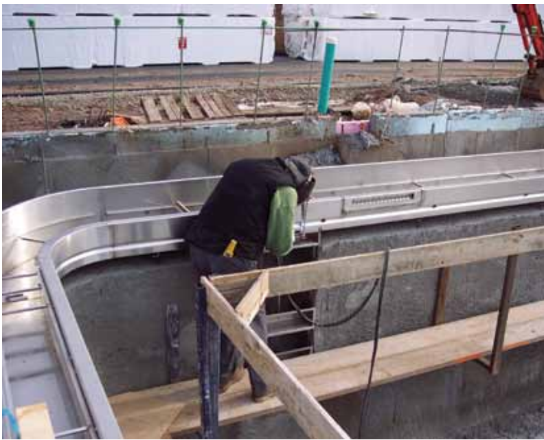
Radius gutter installation above radius shotcrete corner
