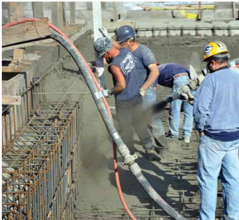
Shotcrete phase of the lap pool
