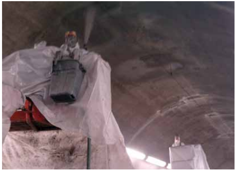
Shotcrete being applied overhead by an ACI Certified Nozzleman
