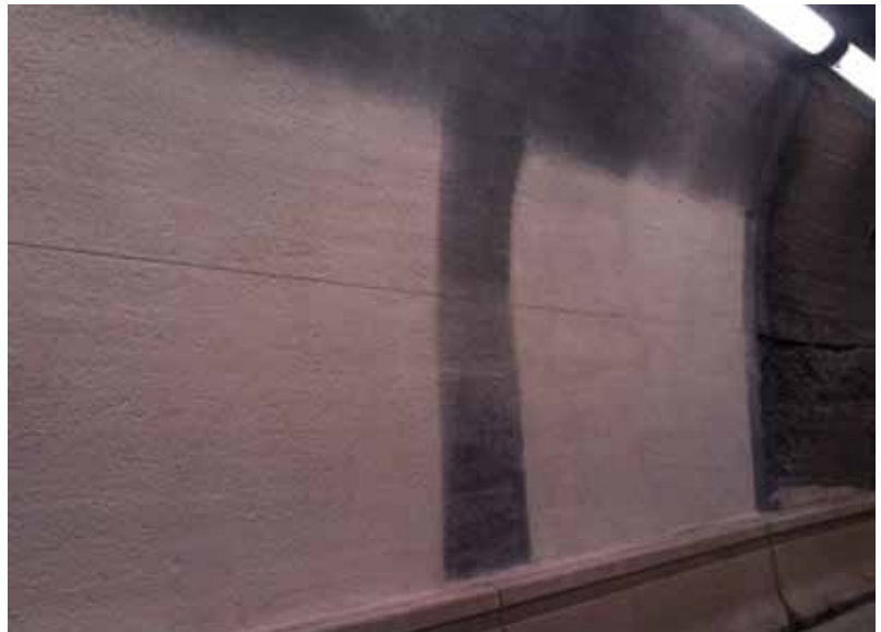
Finished wall with a white to clear curing agent
