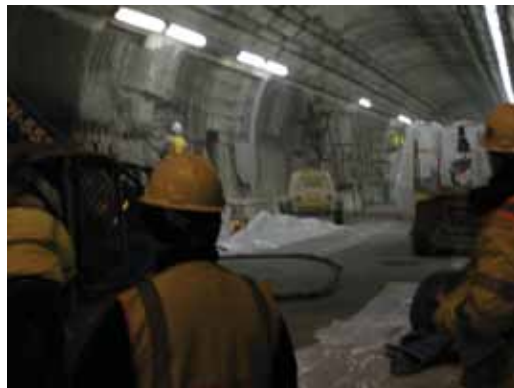
Where necessary, additional reinforcement was installed
