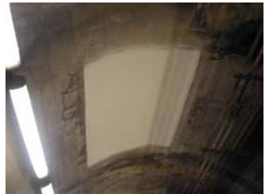
Finished patch on ceiling with white to clear curing agent
