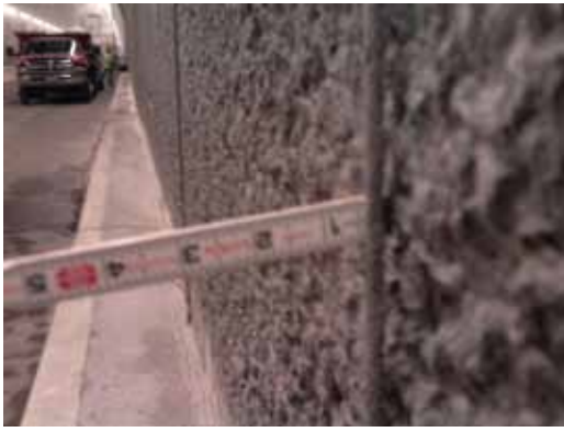
Prepared substrate ready for application of flashcoat
