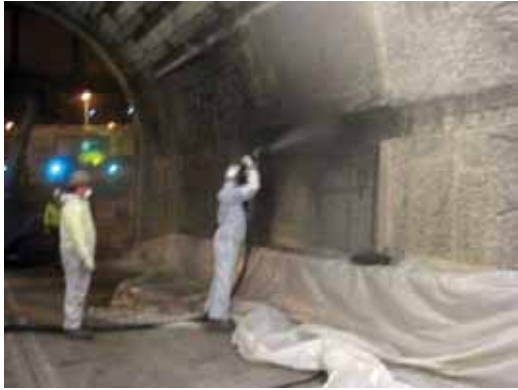
Shotcrete being applied vertically by an ACI Certified Nozzleman
