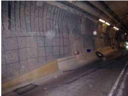
Prior to material installation, the substrate was prepared using hydrodemolition
