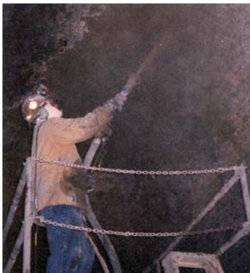
Nozzling performed from mobile scaffolding
