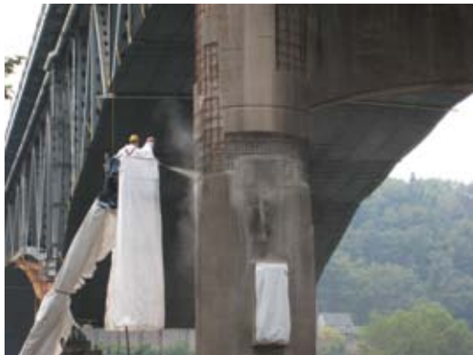
Shotcrete applied at full depth over reinforcing bar and mesh
