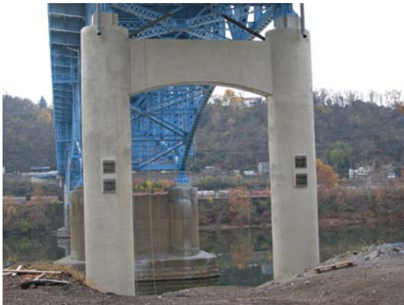
Piers after application of an epoxy coating
