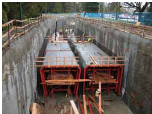
Fig. 7: Side-by-side forms being set
