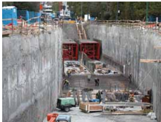
Fig. 6: Side-by-side forms in place, with slab being prepared ahead
