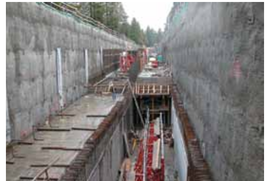
Fig. 9: Rollover section—start of tunnels transitioning to stacked
