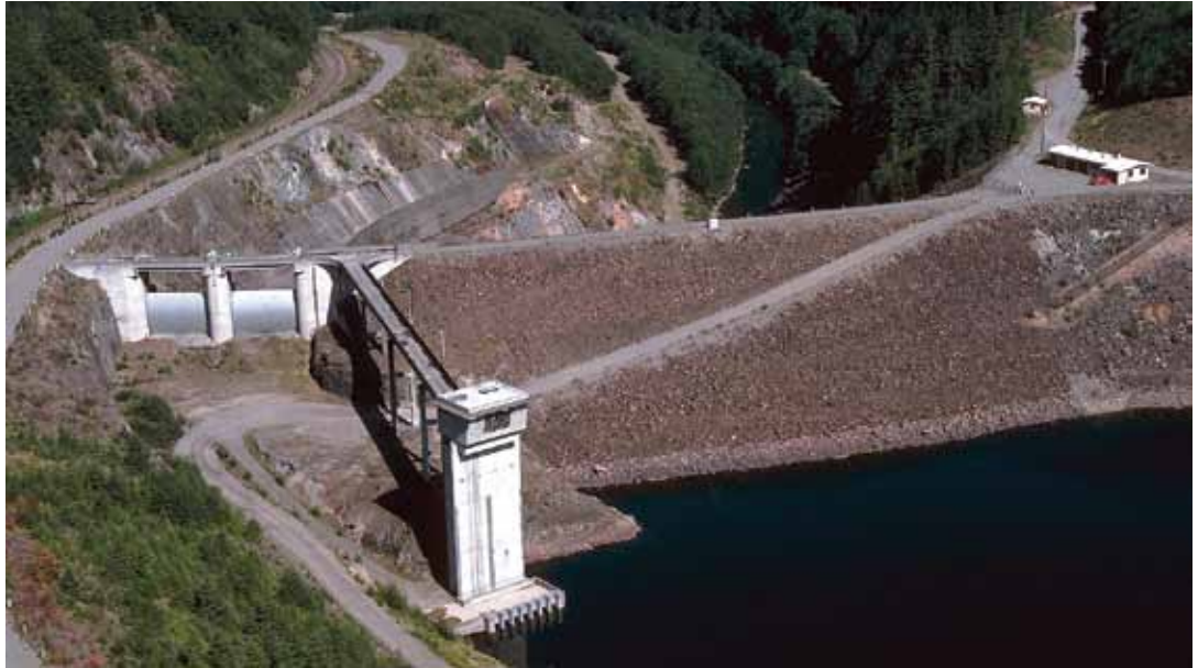
Howard A. Hanson Dam, 1990s Courtesy U.S. Army Corps of Engineers
