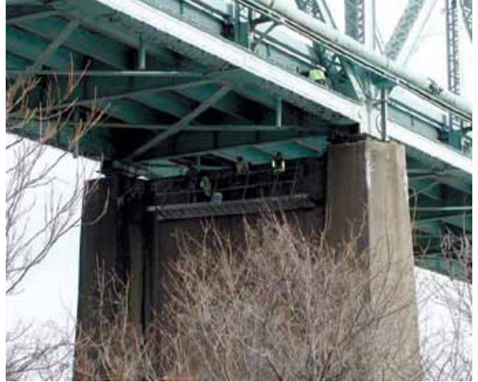
Rigging setup for access to bridge pier
