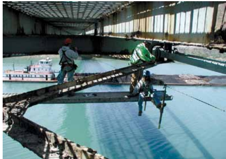
Cable rigging under bridge super-structure
